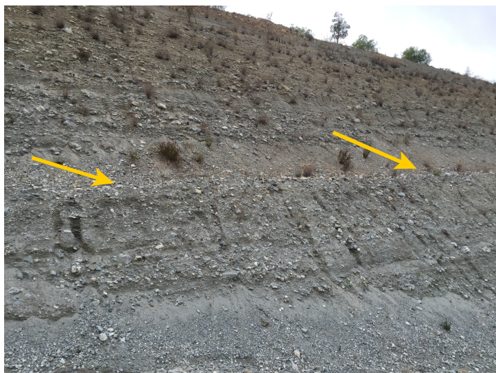
Photo 2: West Pit cut slope and partially buried bench (arrows), view southwest. Incipient rills and general wind/water deflation of the surface are beginning to become more visible. Coarse gravel and cobble clasts stand out in relief. Talus aprons cover parts of the bench and the slope toe along the descending pit haul road. Buckwheat and other perennial scrub species are also becoming established as volunteer vegetation. Height of slope in this view is ~60 feet.
