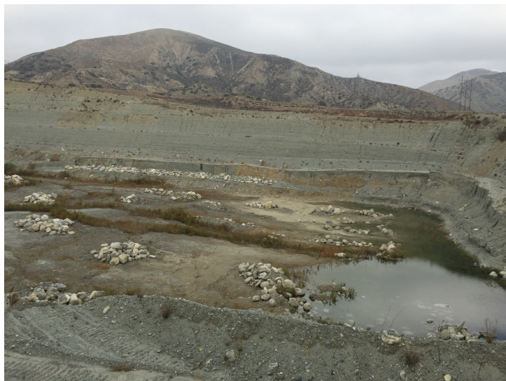
Photo 1: West Pit north-facing overview from the southeastern haul road. Rising-water conditions have remained essentially unchanged in last year. Most flows daylight near the left edge of image and collect in the pond at the eastern edge of the pit floor. Some added volunteer vegetation is apparent along small channels. View area is within permitted vested area. Scale can be judged by stockpiled boulders, most of which are 5-7+ feet in diameter. No mining or reclamation activity was started or observed in the West Pit. Haul road vehicle access is currently blocked by low soil berms.
