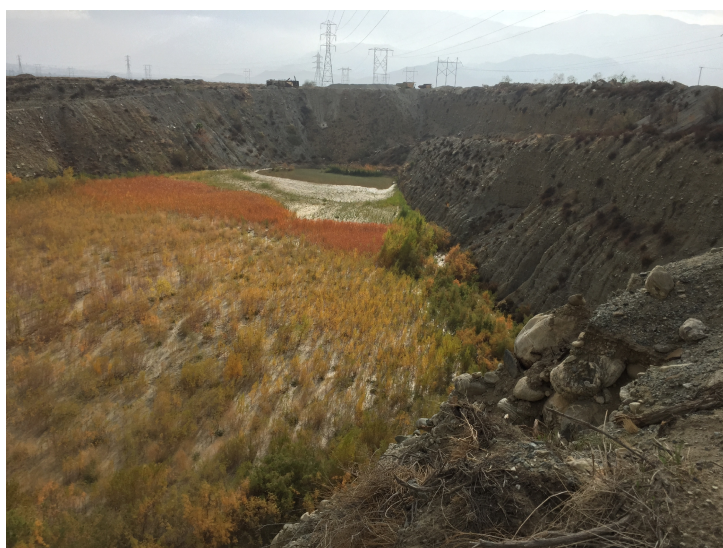
Photo 3: East Pit view to southeast, with wash-water pond and sediment-filled excavation. Except for some rise in the sediment levels, no major changes have occurred in the East Pit. SCE easement passes parallel to the right-side highwall and abandoned haul road. Some slope flattening was reportedly done in 2015 by the operator near the left side of the image. The slope is primarily loose talus. Other, near-vertical brow slopes (out of view) first reported in 2013-2014 were observed to be unchanged but remain for future reclamation tasks.
