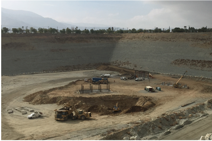
Photo 3: South Pit construction activity, view toward southwestern corner. Foundations and column erections were apparent in three locations, while excavation work for future processing machinery was proceeding in foreground. The construction was reported to be in preparation for relocation of the main rock plant. Some parts of the latter had already been dismantled and were in storage next to the “West Pit extension” pit. Information from the City of Banning indicated the pictured construction was halted by a stop-work order two days after the image date of 12-12-16. Rock plant relocation is an element of the September 19, 2016 MOU between the City and mine operator; however, the amended Mining and Reclamation Plan is incomplete and not yet an approved document. The as-built plant improvements are located in a slightly different part of the pit versus early versions of the amended Plan.
