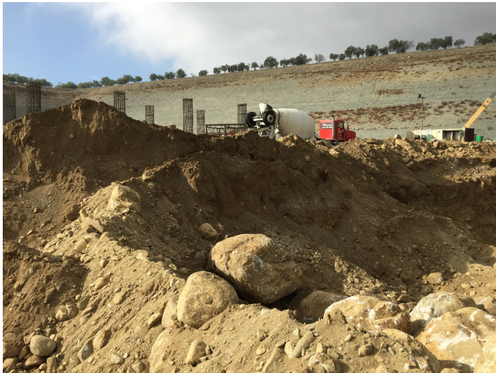
Photo 4: Closer view of under-construction rock plant relocation site, view southwest. Yellowish tones to the excavated alluvial sediments indicate greater geologic age and higher fines contents than most mined sediments. Transit mix truck arrived during the inspection visit.
